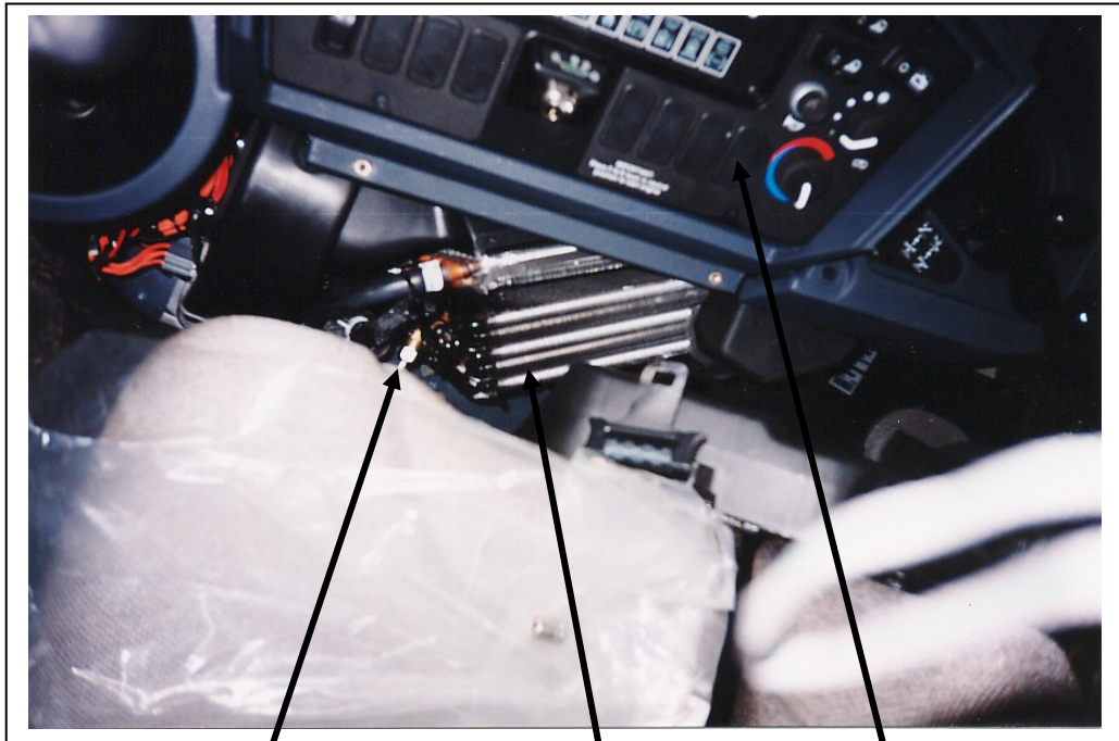
5/16" 90o fitting at expansion valve
